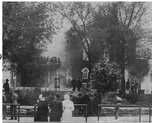
This Picture Was Taken May 7, 1919, While the Court House Was Being Consumed by Fire
