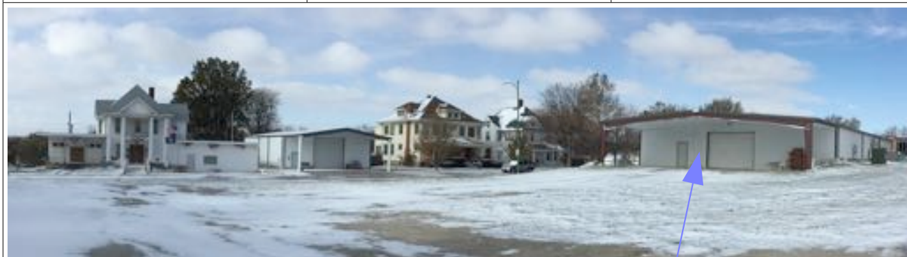
AG II Building Completed September, 2019 !!
